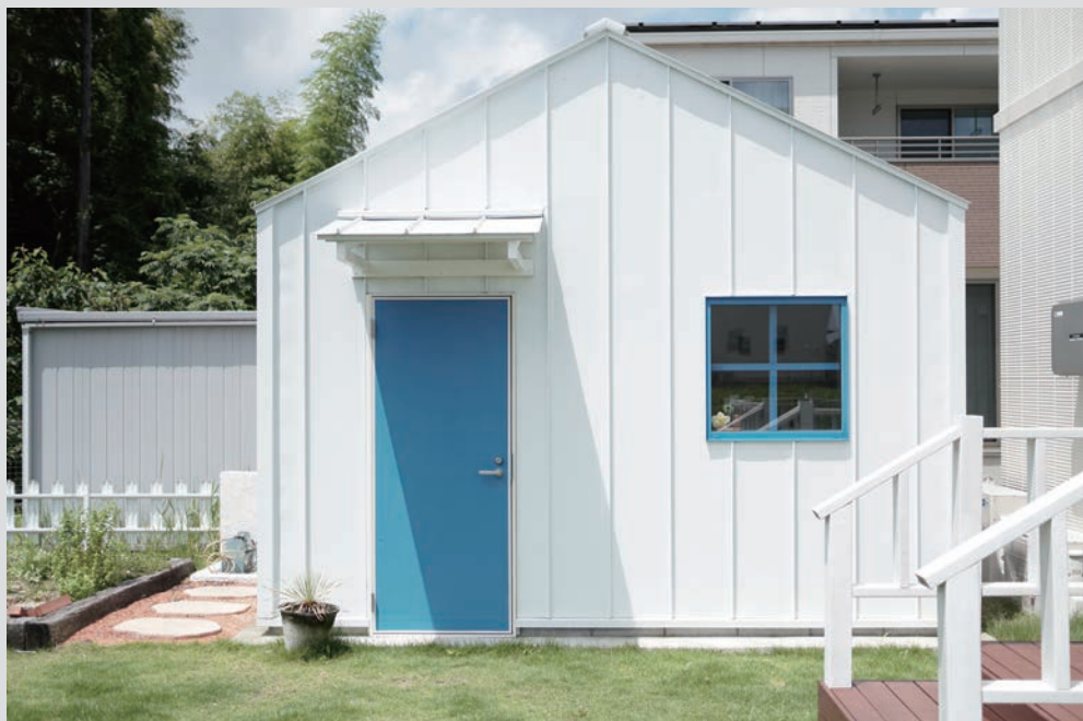
施工：MOUNTAIN HIGH
